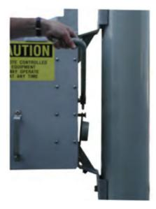
2. Remove the padlock and rotate the collar out of the way. Place handle over the exposed shaft and insert interlock pin. Switch is now operated like any manual switch.
