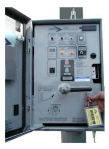
1. Remove the interlock pin from the front panel and insert it into the output shaft and padlock in place. Decouple the operator.
