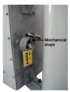
3. For a clearance, repeat step 1, and place interlock pin through shaft. Replace collar to capture the interlock pin at a mechanical stop. Padlock collar for final clearance point
